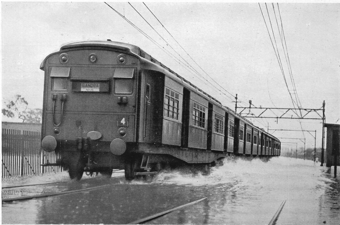
These two views are of interest in showing the routine operation of the first electrified line in India. Suitable design of the motors prevented any interruption to the service by the monsoon floods.
