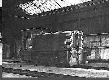
One of the two Ruston & Hornsby 165hp 0-4-0 diesel shunters built for BR in 1956 - No.D2958 (ex-No.11508) in BR green livery at Stratford MPD in July 1967.
