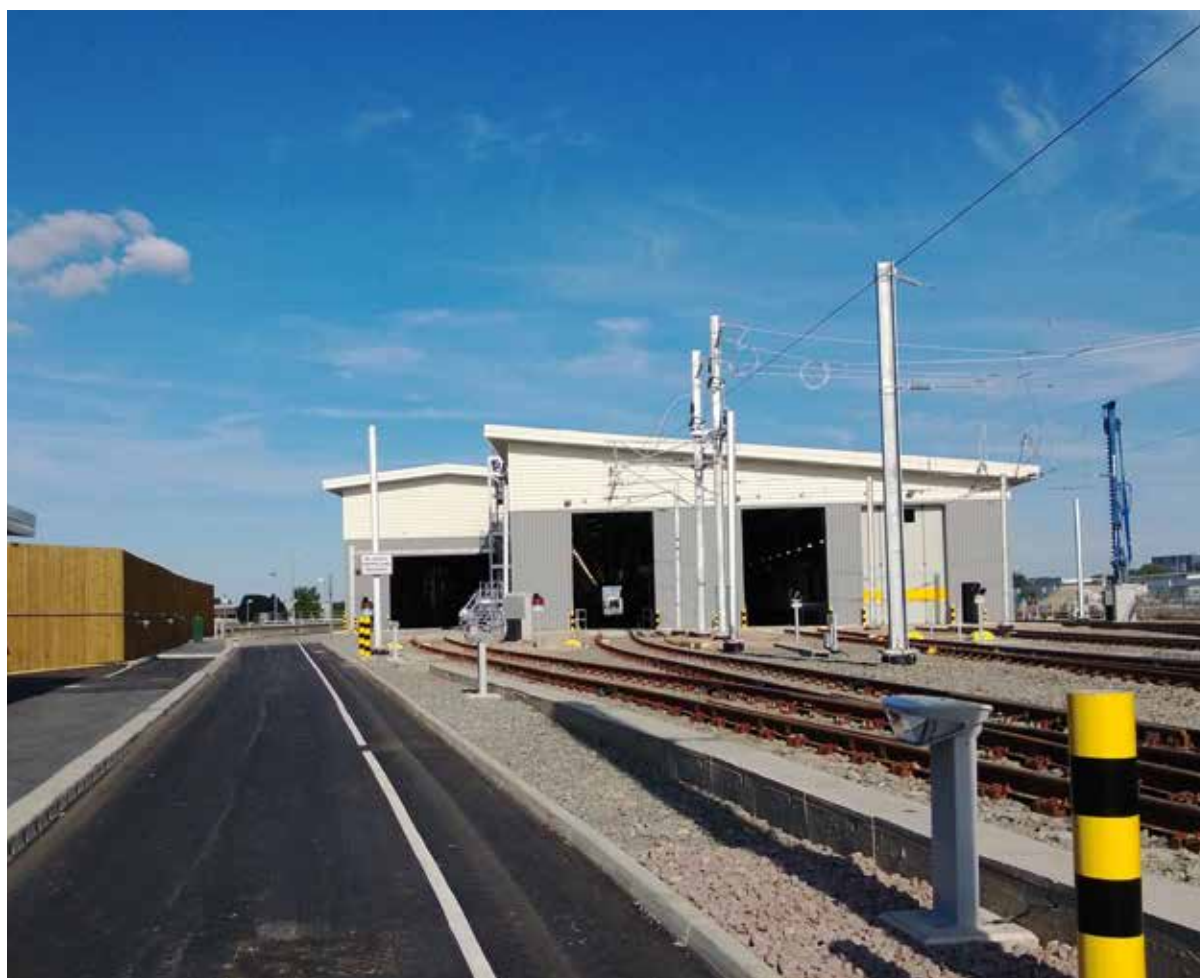
FGW's new maintenance depot at Reading, opened in 2013 as part of the Reading Station Area Redevelopment capacity upgrade
